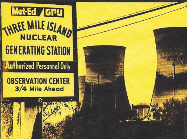
APPROACHING COLD SHUTDOWN - Technicians worked to achieve a cold shutdown following a near-crisis that reportedly allowed radioactive steam to leak into the air surrounding a reactor at the Three Mile Island plant in Pennsylvania.
