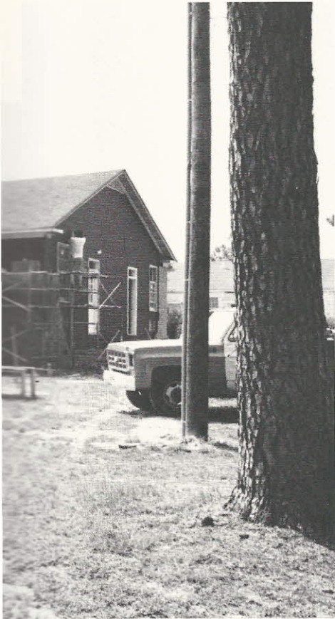
with its new wing nears completion.
