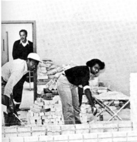
ng bricks are Deneen Adams and Kevin Williams .
