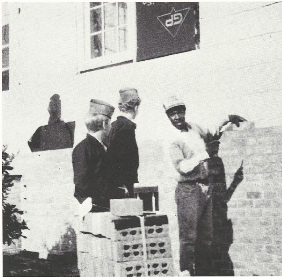
. . . Preston Stout and David Doerr observing a mason at work on restoring the fire-damaged classroom building.
