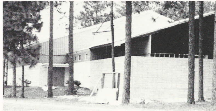
The gym addition underway, its completion weeks away.
