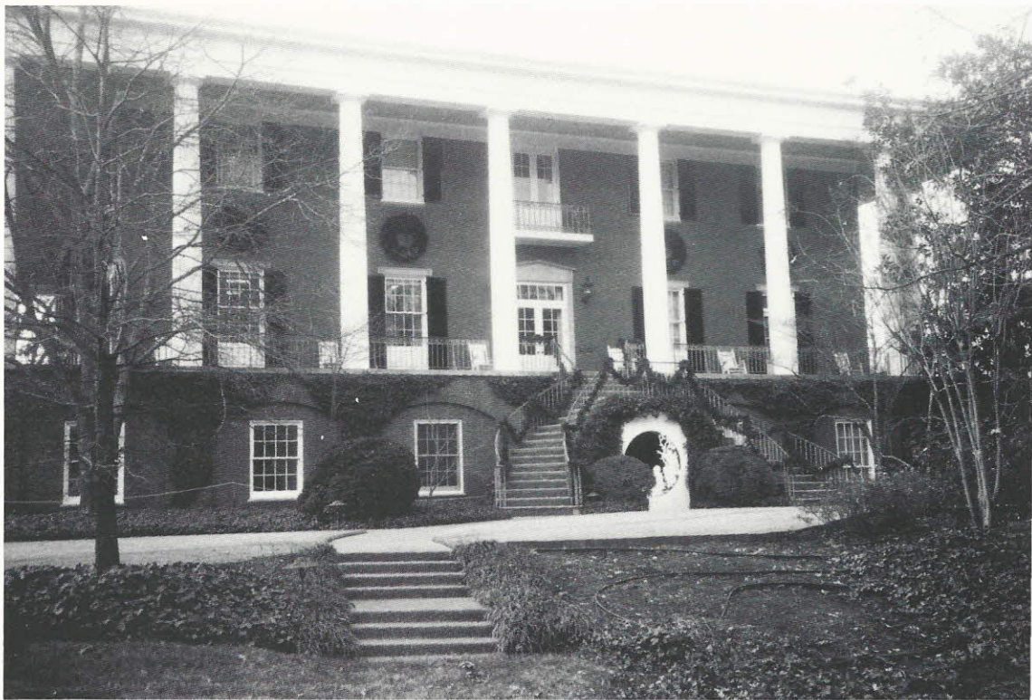
Over the years, Georgia's chief executive has been housed in several locations. Shown here is a wing of the present mansion, which was built in 1975.
