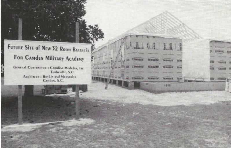
New Barracks: From a spot on the ground to an impressively large structure gradually taking shape, the new barracks through "cellular growth" will eventually become a comfortable building of 12,000 square feet.
