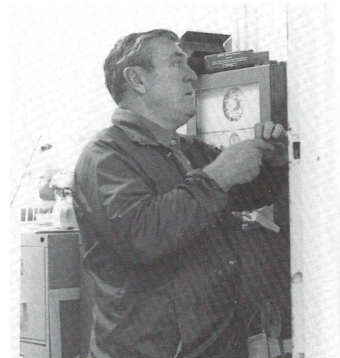
Mr. Harmon works on the intercom system in the office.
